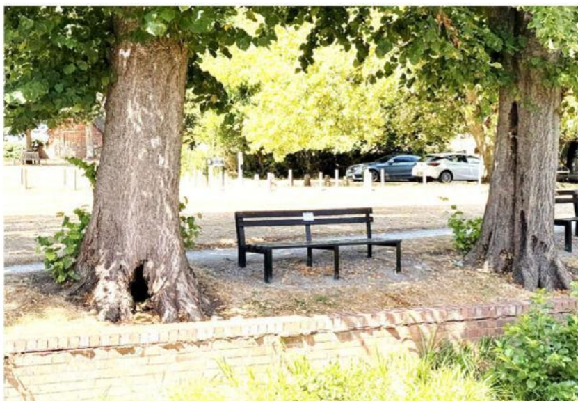
Photograph 4: Showing the decayed trunks of previously condemned trees 824 and 825.
