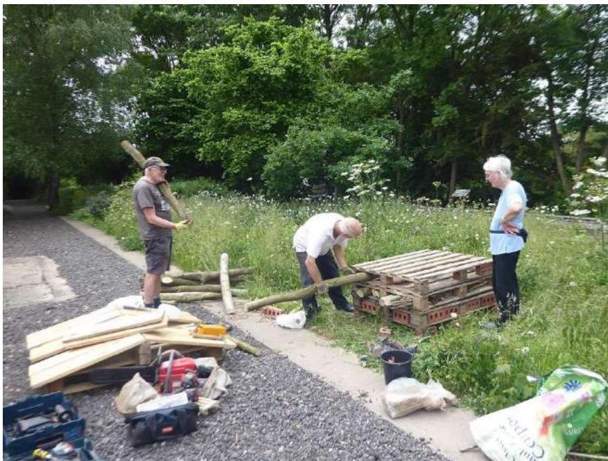
Above: Building the Bug Hotel 2021
